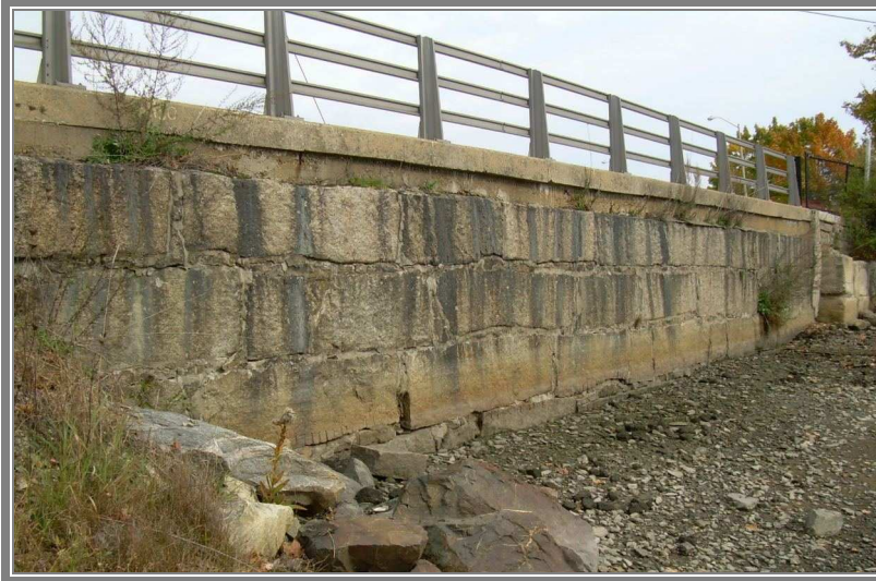
PHOTO 26 Maplewood Ave south wall east.
