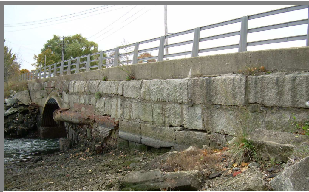
PHOTO 20 Maplewood Ave north wall – note deterioration at penetrations.
