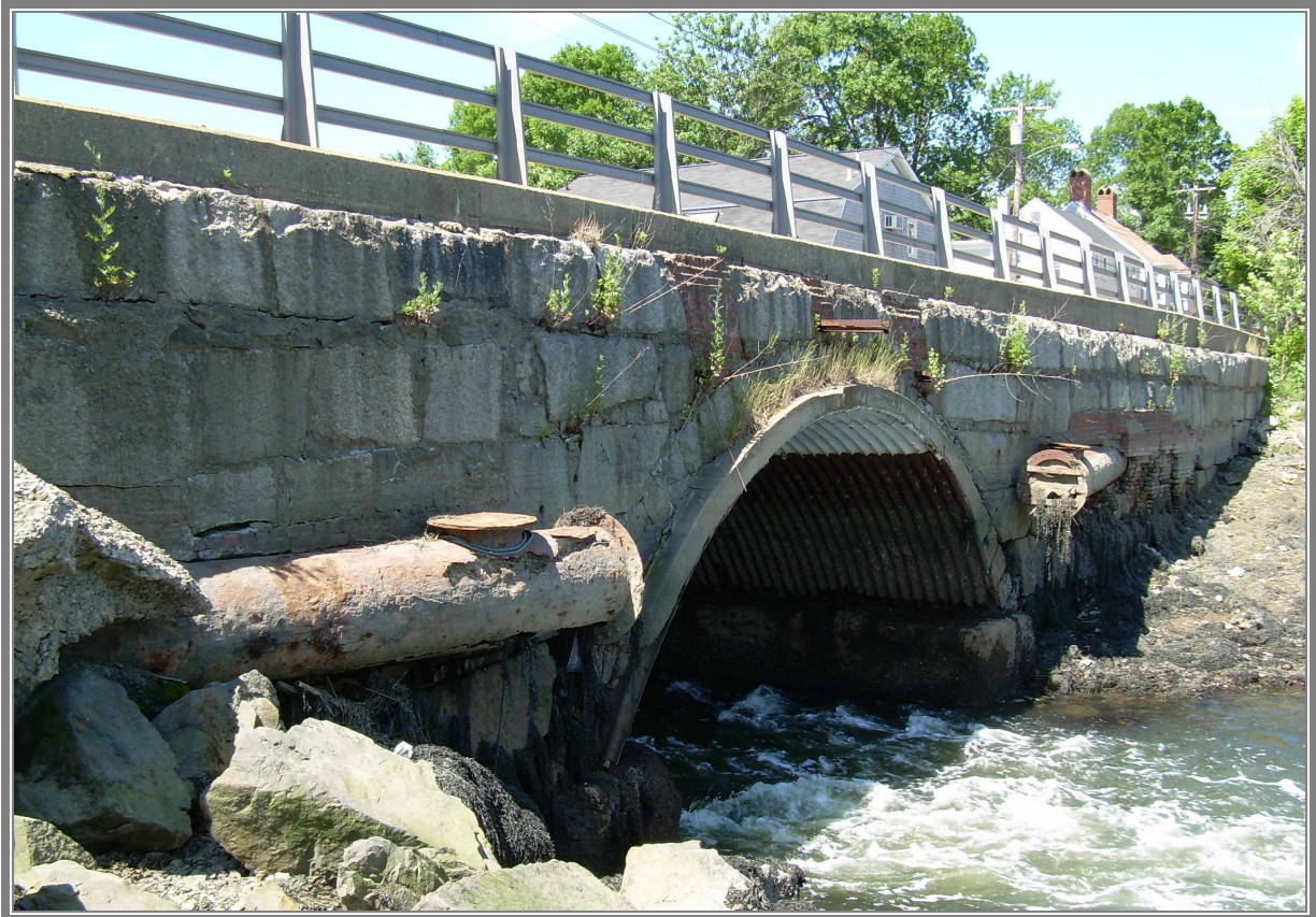
PHOTO 19 Maplewood Ave north wall – note abandoned sewer line penetrations.
