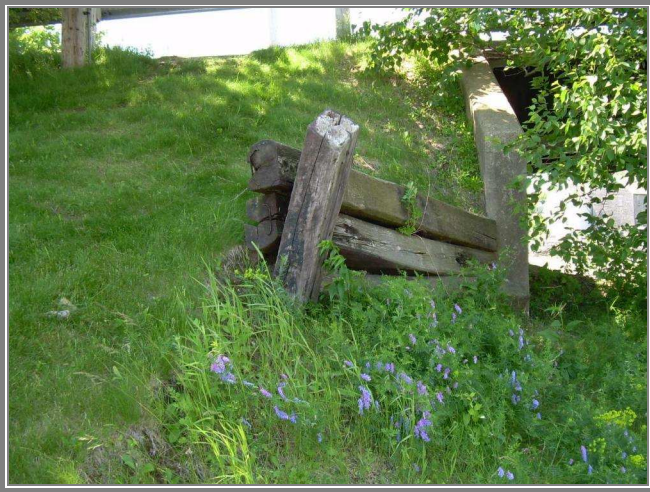
PHOTO 15 Pierce Island Bridge north approach wall leaning down slope.
