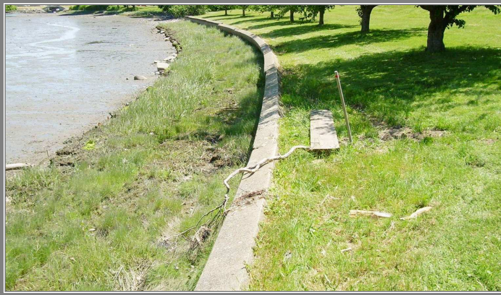
PHOTO 28 South Mill Pond near Police Sta. – note wall rotated offshore.
