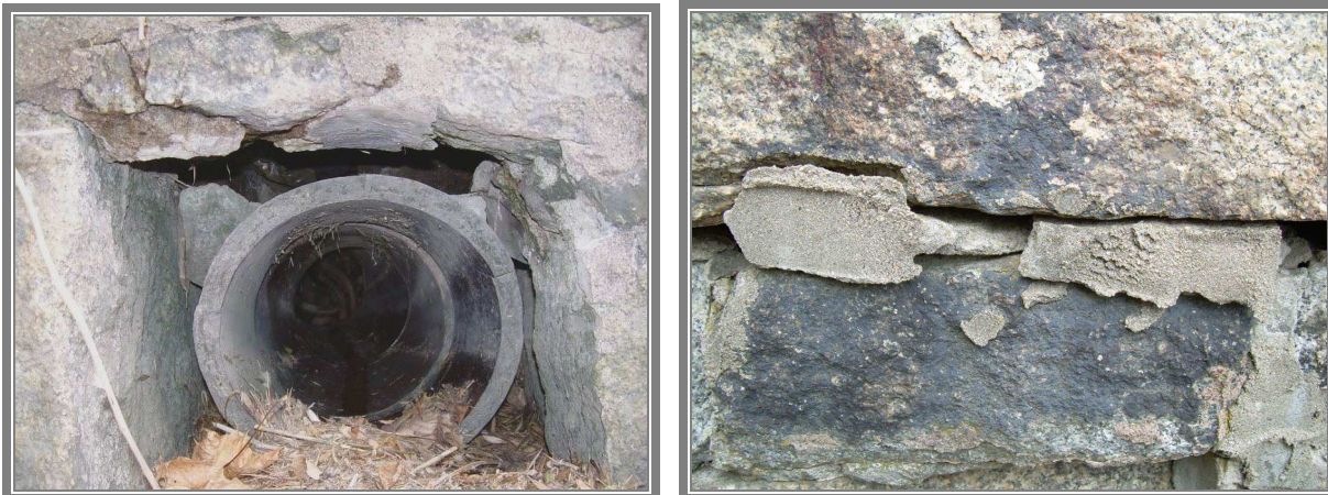
PHOTO 23 & 24 Maplewood Ave south wall west drain outfall & opened joints.
