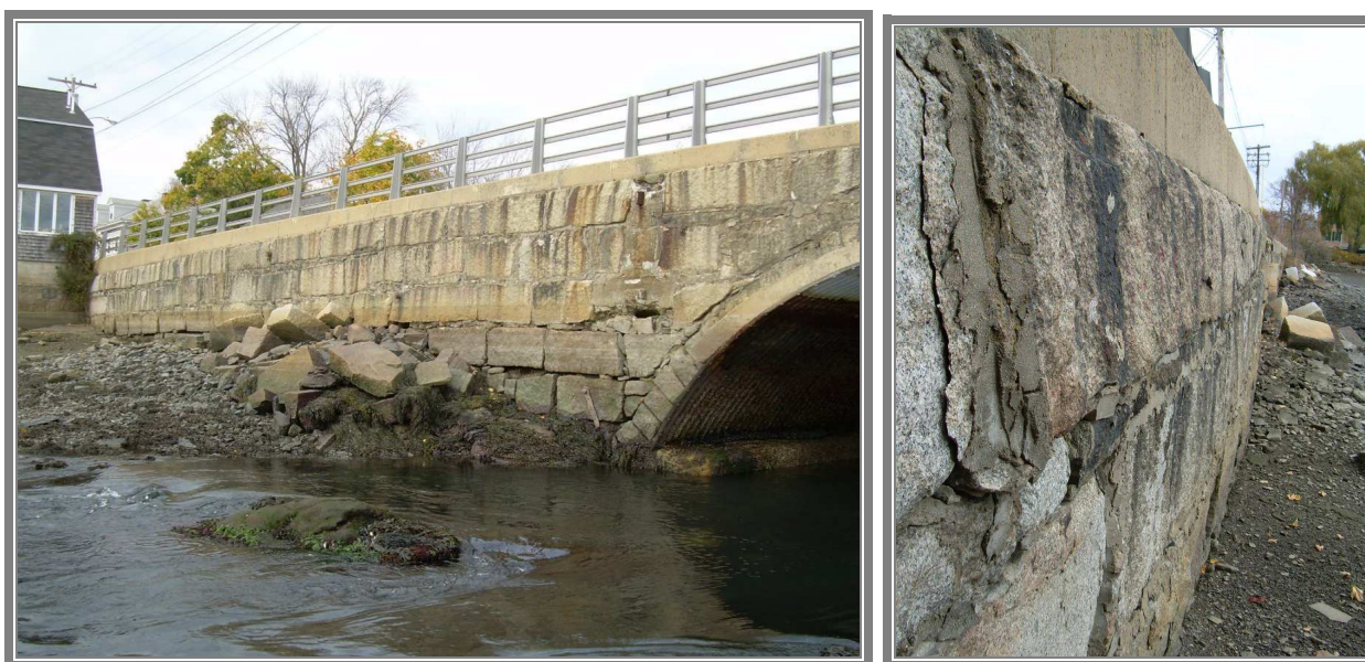
PHOTO 21 & 22 Maplewood Ave south wall west with bulge and opened joints.
