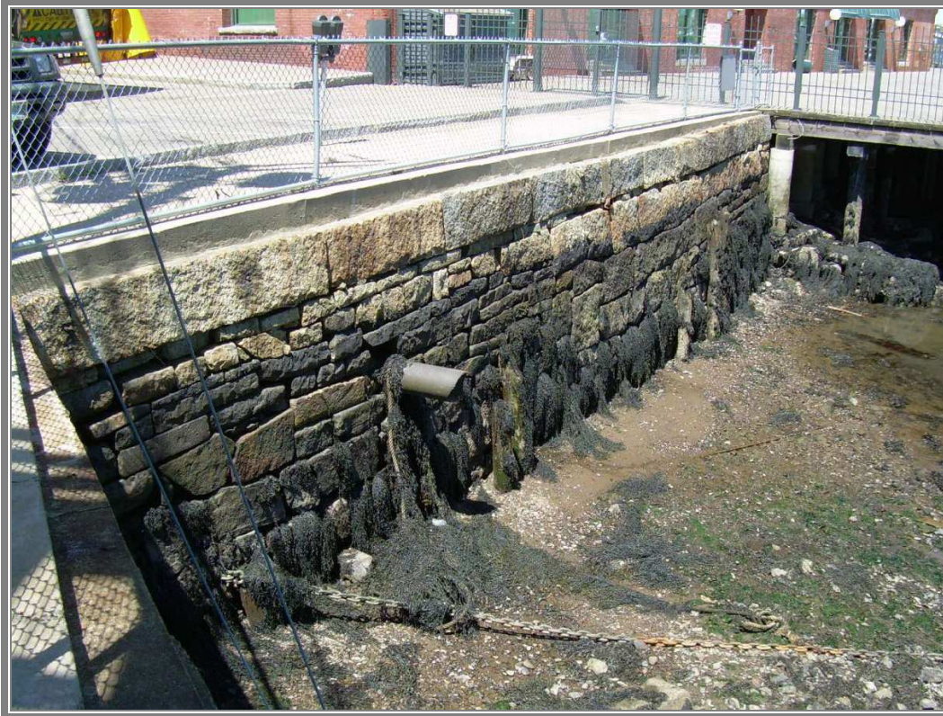
PHOTO 16 Daniel St primary seawall section – note tensioned floating dock mooring chains attached to wall base stones.
