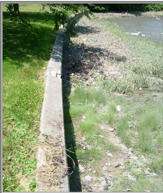
PHOTO 29 South Mill Pond near Police Sta. – west end with wall rotated offshore.
