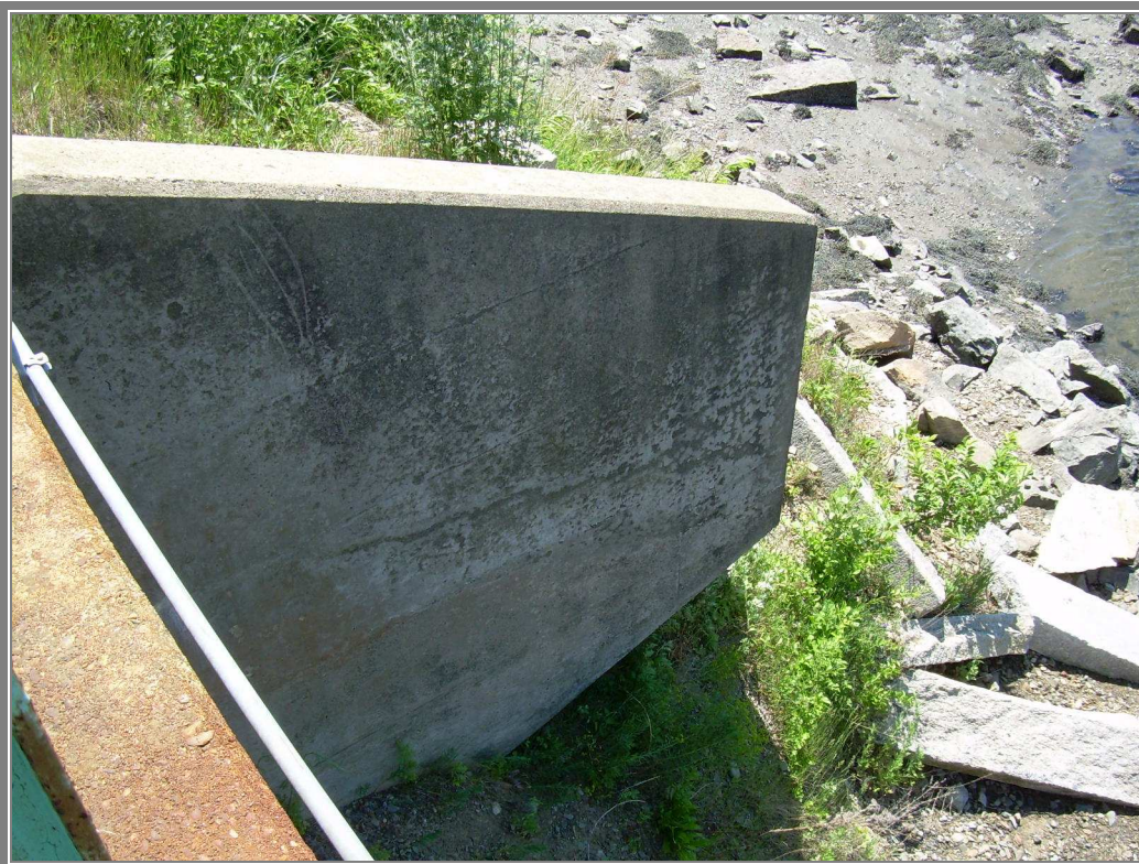
PHOTO 14 Pierce Island Bridge south wingwall undermined by erosion.
