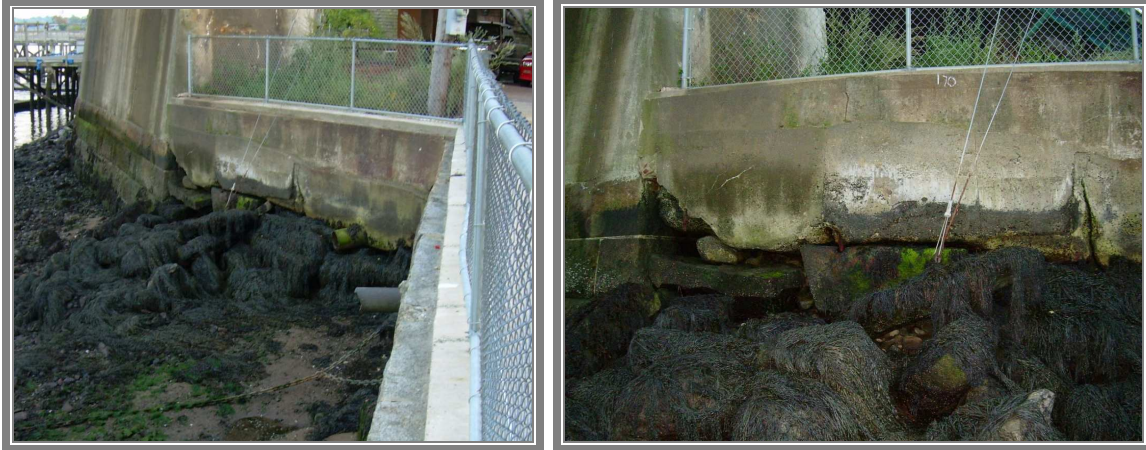
PHOTO 17 & 18 Daniel St end seawall section – note gaps under concrete.
