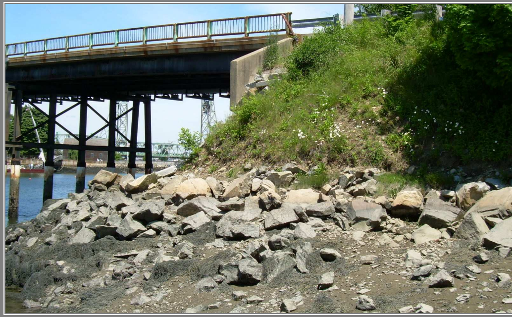
PHOTO 13 Pierce Island Bridge south approach wall (the granite blocks, not the concrete abutment) – note slope erosion above riprap.
