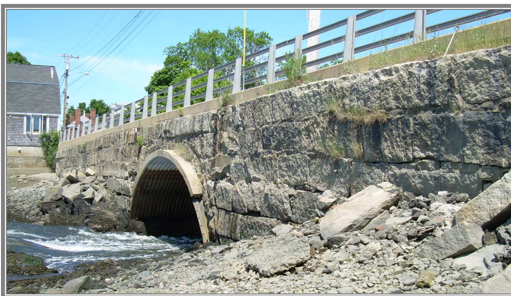
PHOTO 25 Maplewood Ave south wall at culvert.
